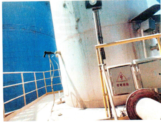
1#线窑尾排气筒 (◎1)
